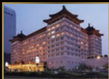
GRAND PARK XIAN The best South Gate location, overlooking the majestic City Wall
