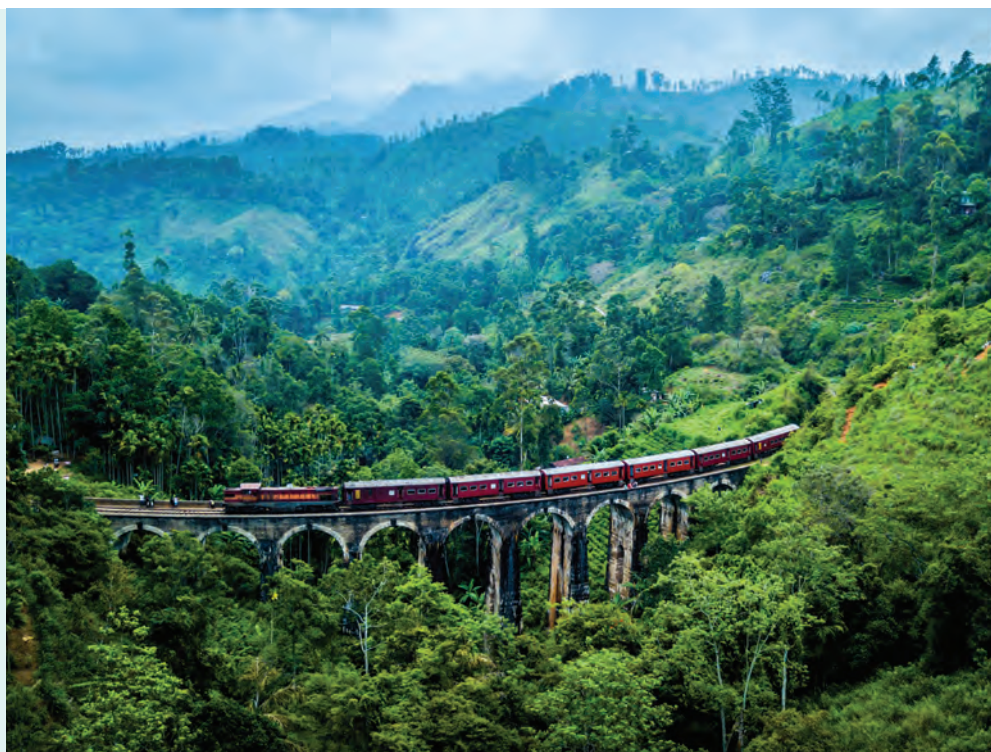
Nine Arches Bridge in Ella
